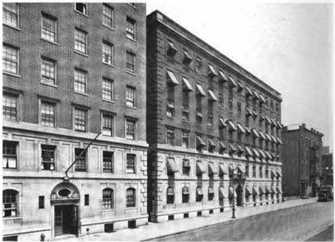
FIG. 103. GENERAL VIEW—APARTMENT BUILDING AT 305 WEST 45TH STREET, NEW YORK CITY. Evarts Tracy, Architect.
