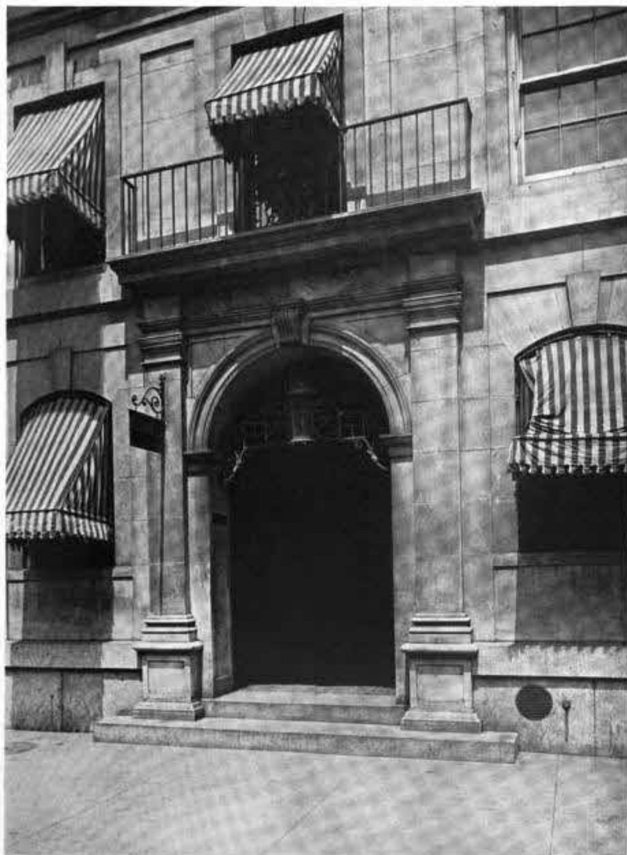
FIG. 104. DETAIL OF DOORWAY—APARTMENT BUILDING AT 305 WEST 45TH STREET, NEW YORK CITY. EVARTS TRACY, ARCHITECT.
